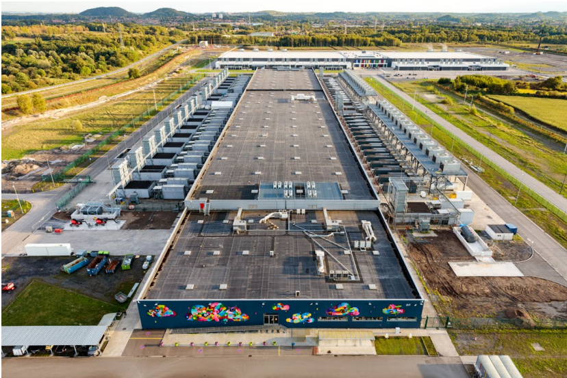
Figure 1.7: Example of a Hyperscale data center of Google in St. Ghislain, Belgium. Since the completion of the first DC in 2010 in St. Ghislain, Google has extended the site with two new DCs and has announced a fourth DC in June 2019 with an investment of 600 million USD [12].
