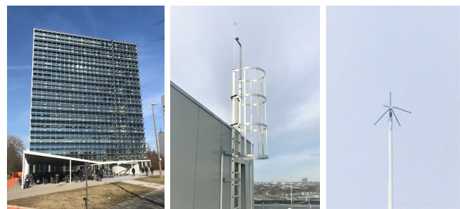
Fig. 1: Base station antenna (right) on top of the access ladder (middle) to the uppermost roof portion of the office building (left) located at marker A.
