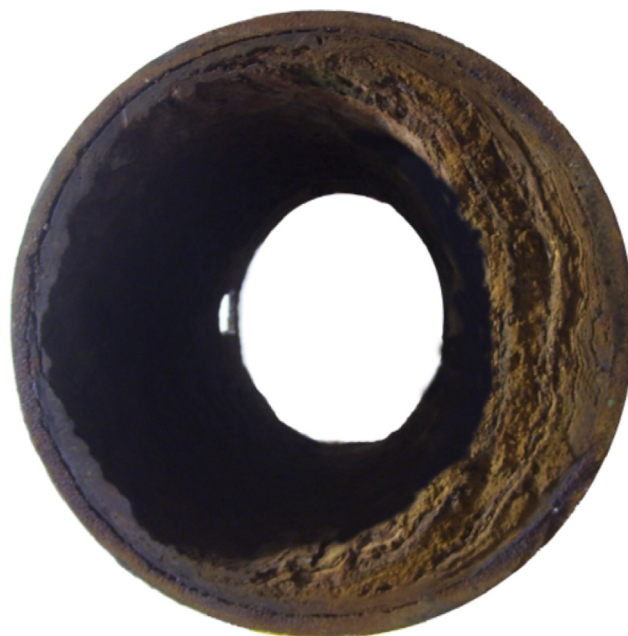
Fig. 1 A sample of scale layer formed in an oil pipeline [25].
