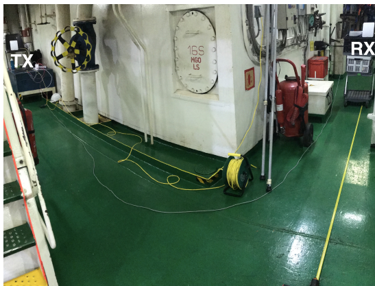
(a) Receiver is behind the corner in engine room
