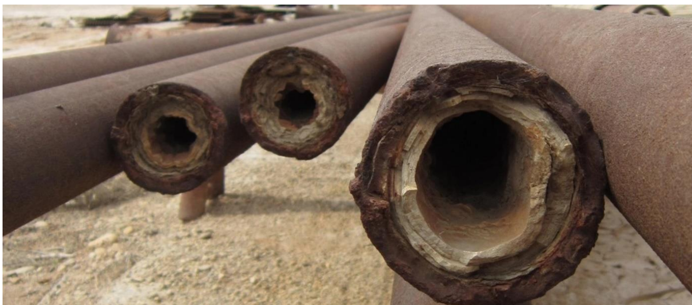
Figure 1. An example of scale deposition in few pipes.
