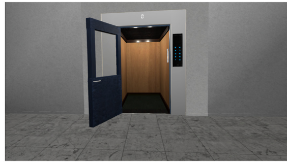
(b) Old elevator with a hinged door featuring a window. The buttons are located on the outside.
