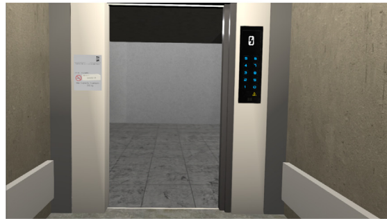
(c) Service elevator with a one-sided sliding door.
