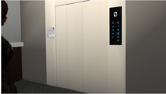
(a) Modern elevator with two-sided sliding doors.
