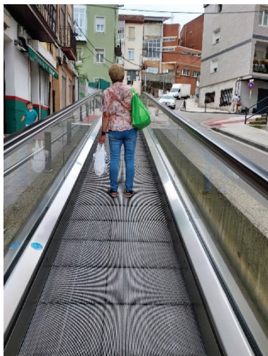
Picture 2. Urra S. (2021), "Mechanical ramps installed in the city of Santander to solve accessibility issues".
