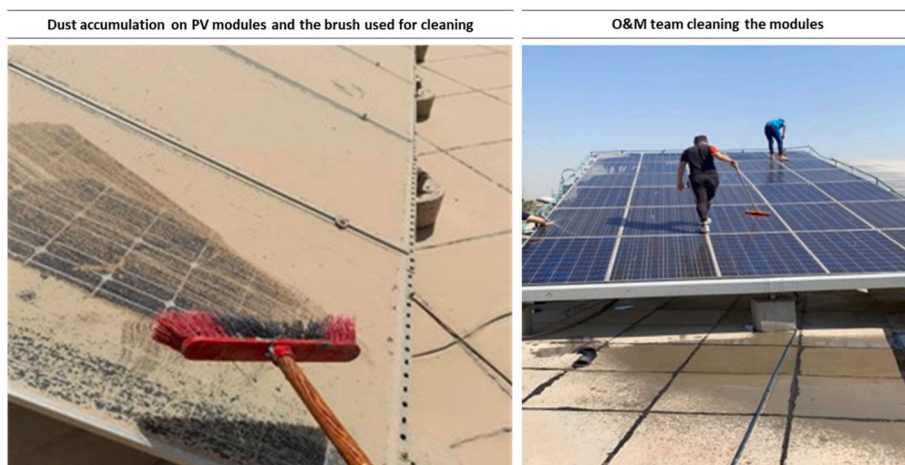
Fig. 4. Dust accumulation on PV modules installed in Iraq and the cleaning process currently used.
